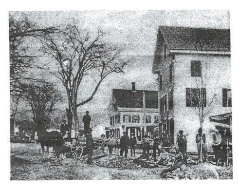
This picture shows the crew of the Water Precinct digging up a piece of pipe near the center of Freedom Village. In those days (about 1913) the pipes were made of wood, and the way leaks were discovered was finding a rivulet of water somewhere on the road. Records of the location of the new, metal pipes used to replace the rotting wood were incomplete so no map could let the commissioners know just how much old pipe was left.
